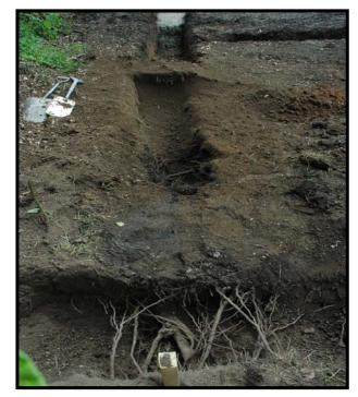
Where it becomes necessary to excavate a trench close to or under the canopy of a tree, these tools can be used to expose roots that may then be either bent out the way of the trenching work or cut back using target pruning. This reduces the stress caused to trees by preventing roots being ripped out the ground by a mechanical excavator, therefore prolonging the trees life expectancy and enabling the retention of trees that may otherwise have been removed.
